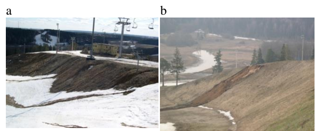
Fig. 1. Monitoring data of RSC «Sorochany»: a – one of the hills before woodland conservancy work (03.2006), b – unexpected landslide (04.2008).
