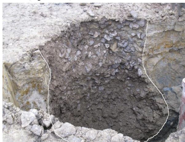
Fig. 3. Visual inspection (excavation) of the column.
