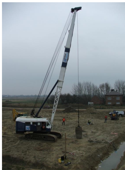
Fig. 2. Process of the stone column formation.
