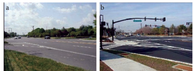
Fig. 6. Safety enhancements at intersections: a – unsigned, open mode; b – textured crosswalks and expanded islands
