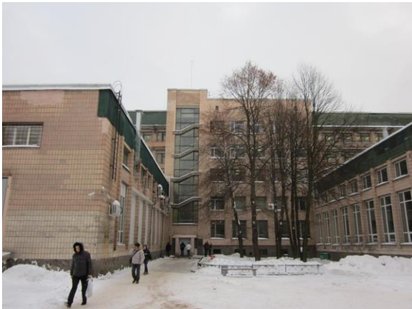
Fig. 3. "Hydrotechnical building-2" at the campus of SPbSTU.
