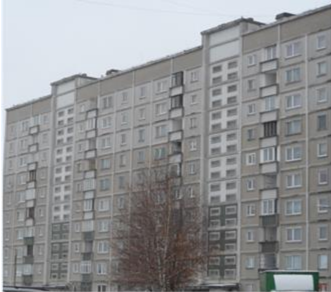
Fig. 9. Residential house on Valdeku Street 51, Riga [7].
